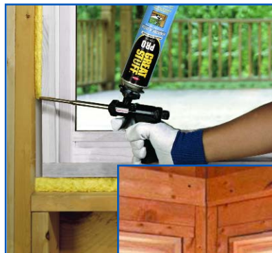
Unlike fiberglass insulation, GREAT STUFF™ Pro Window & Door resists water intrusion and compresses easily as the frame expands and contracts, while still maintaining an adhesive bond.
