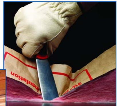
Compressing fiberglass causes it to lose its insulating value. Stuffing fiberglass into the narrow, hard-to-fill gaps surrounding a window or door frame provides limited insulating value but a poor air seal.
