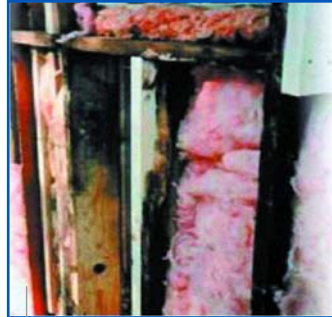
Fiberglass, when wet and compressed, loses a significant portion of its insulative value and over time could serve as a catalyst for mold, mildew and other unwanted bacteria.
